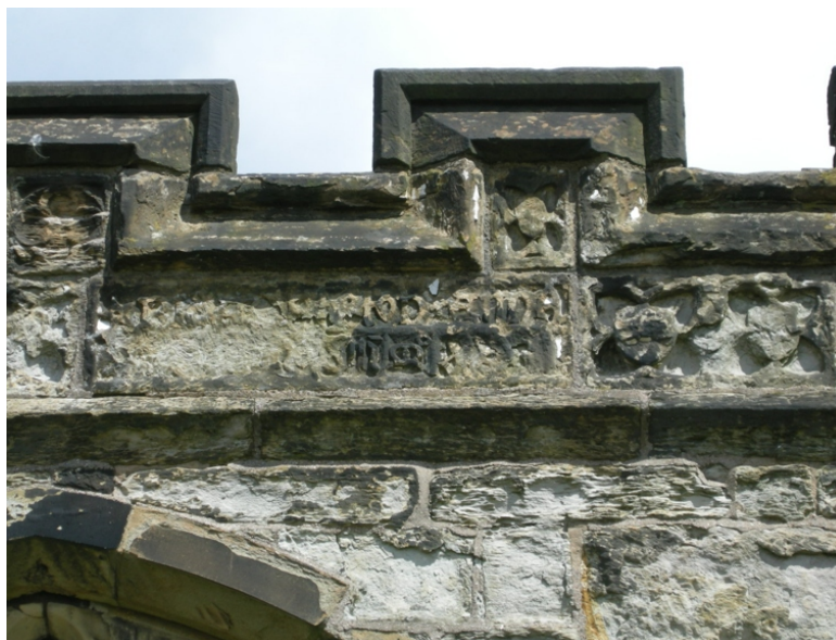
Stone erosion on the south elevation
